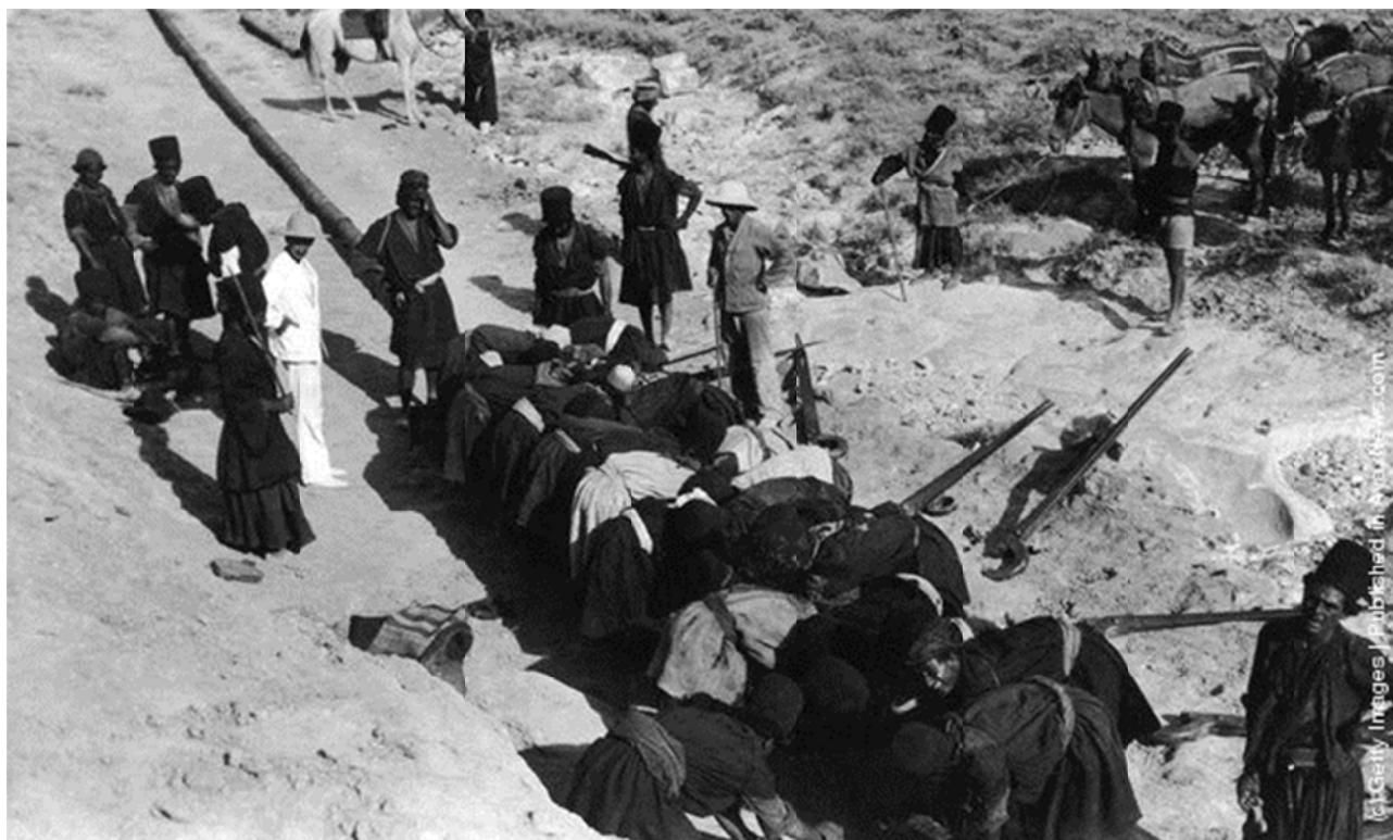
Laying the Anglo-Iranian Oil Company pipeline between Masjid-i-Suleiman and Abadan in Iran, circa 1910. The pipeline was completed in 1911. (Photo by Hulton Archive/Getty Images)
